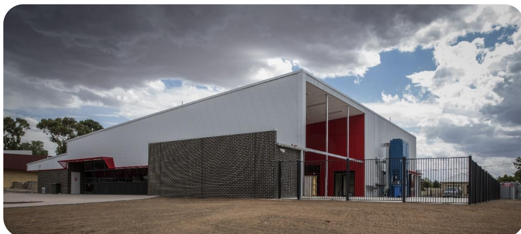
Outside view of the Training and Innovation Hub building
